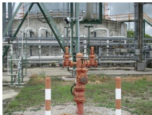
Water Monitor with Remote
