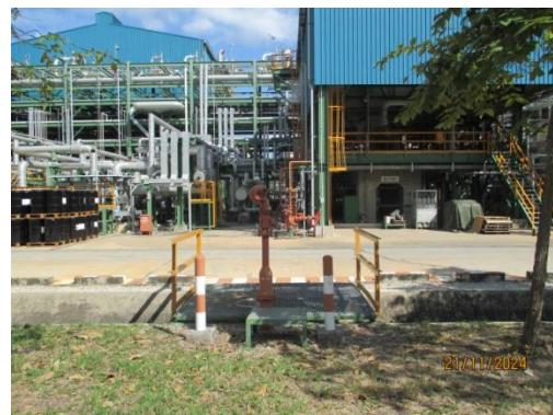
Water Hydrant with Monitor
